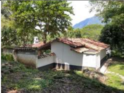
CHIMENEA DOMESTICA N: 5°49'50.21" O: 75°42'17.83"
